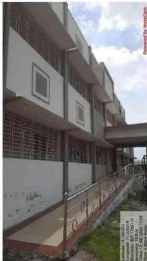
RAMP IN E BLOCK
