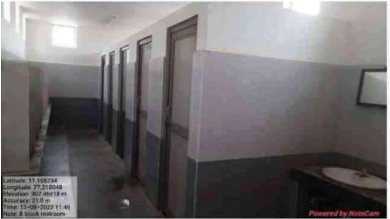
RESTROOM IN B BLOCK
