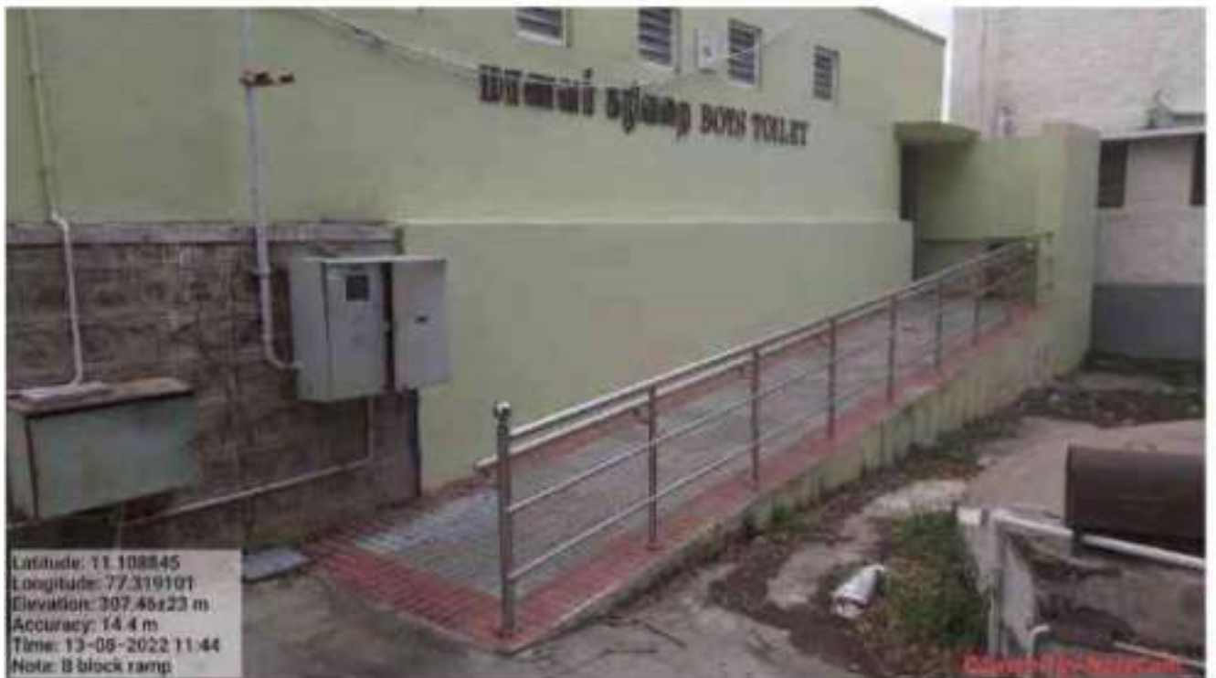
RESTROOM RAMP IN B BLOCK
