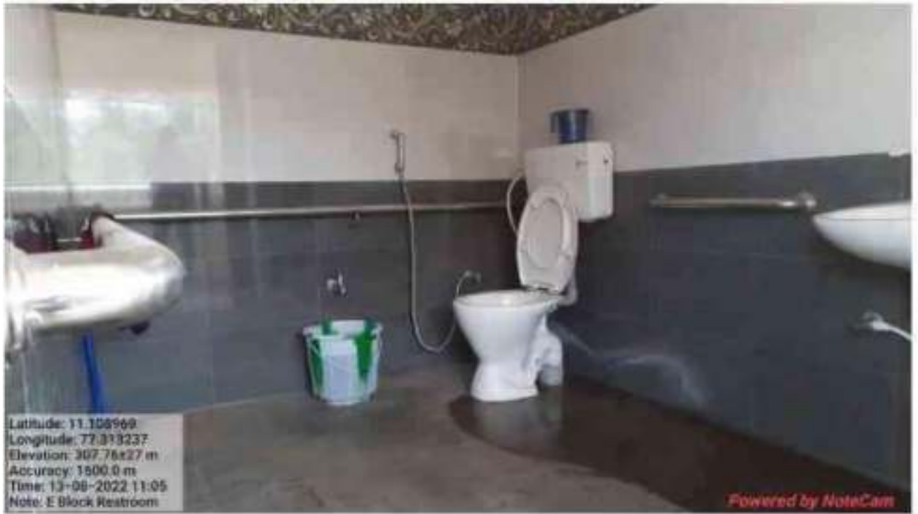
DIVYANGJAN-FRIENDLY RESTROOM IN E BLOCK
