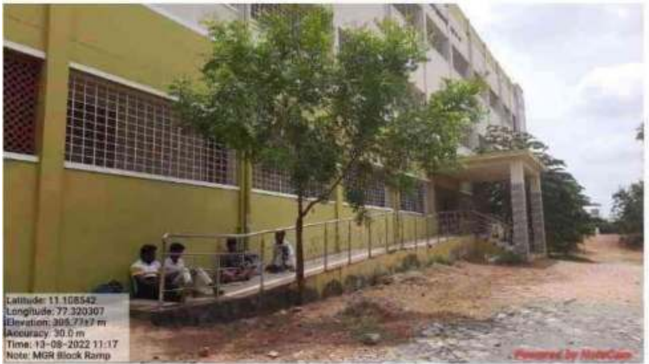
RAMP IN MGR BLOCK
