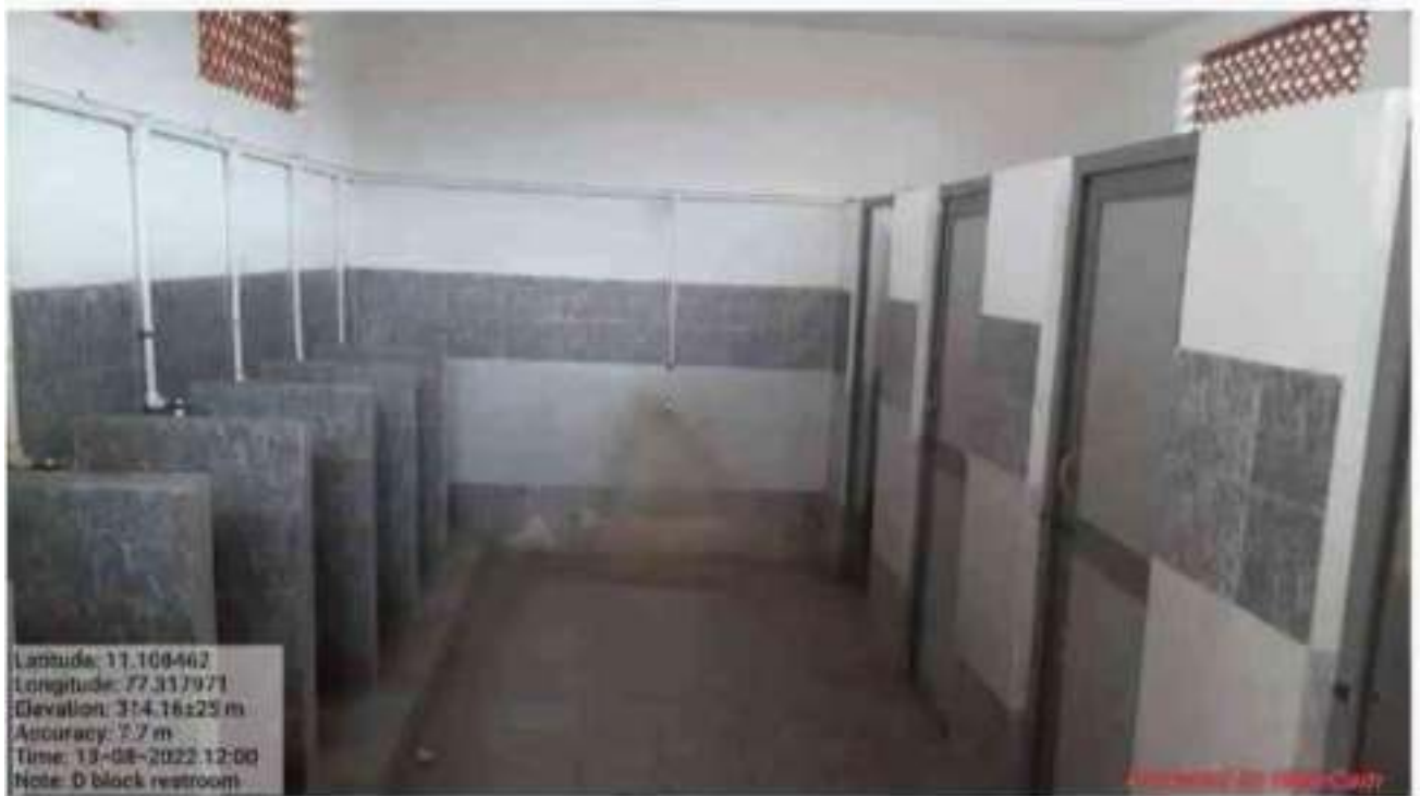
RESTROOM IN D BLOCK.
