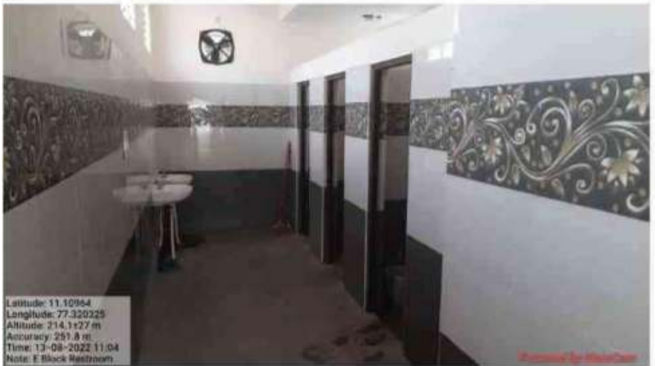
RESTROOM IN E BLOCK
