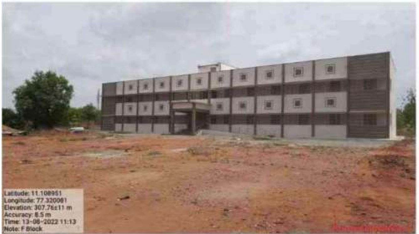
NEWLY CONSTRUCTING F BLOCK
