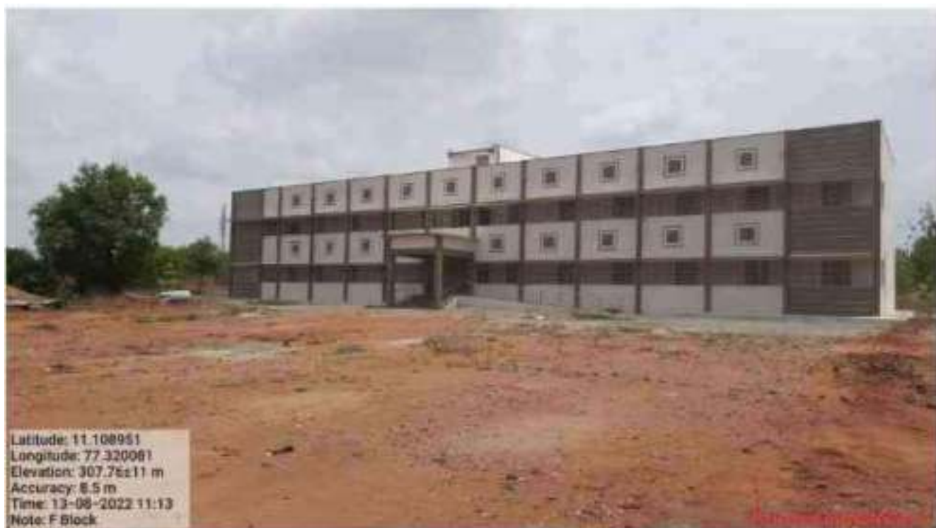
NEWLY CONSTRUCTING F BLOCK
